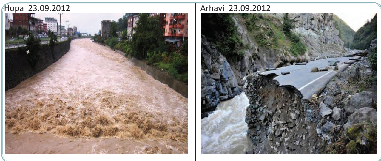
Figure-88 Flash floods in Hopa and Arhavi towns on 23-24 September 2012
