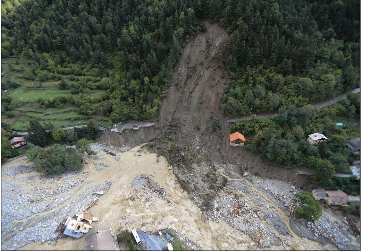
Şekil 42. Fransa-Saint-Martin-Vesubie'de sel ve heyelan hasarı (3 Ekim 2020) ( https://www.theatlantic.com/photo/2020/10/photos-flooding-southeastern-france/616629/ )
